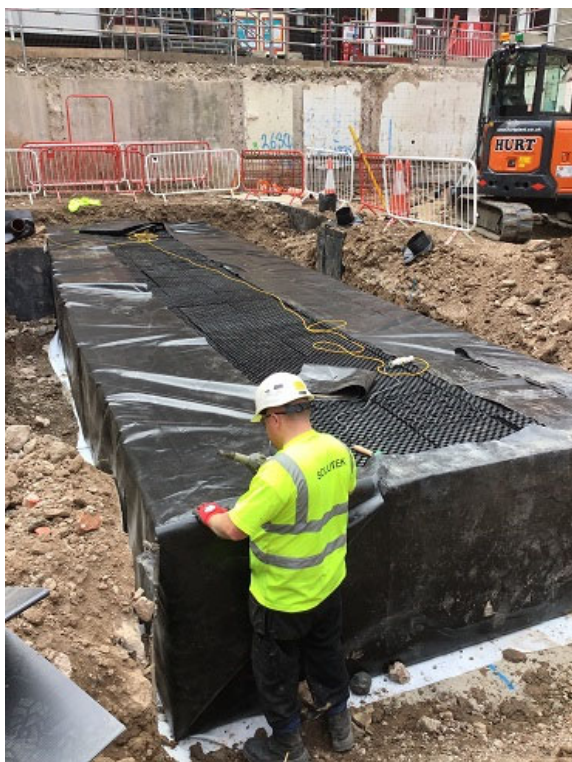
Photograph 2 – Attenuation Tank Installation
