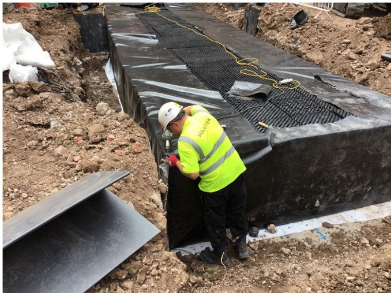
Photograph 1 – Attenuation Tank Installation
