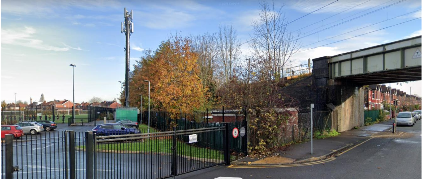
View from Lytham Road looking towards the existing mast to be replaced
