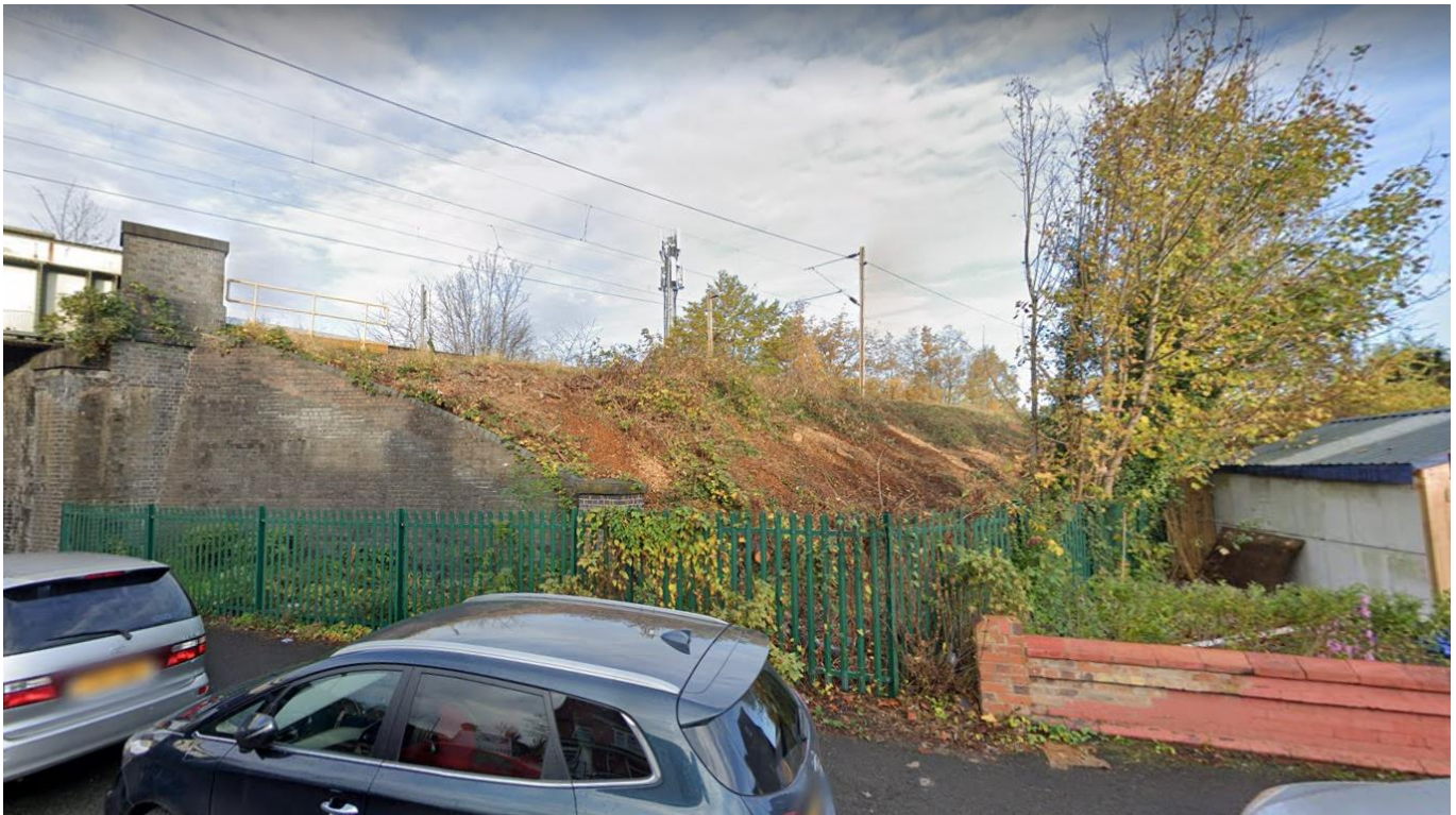
View from the eastern side of the Lytham Road rail bridge looking north-west with cleared embankment centre
