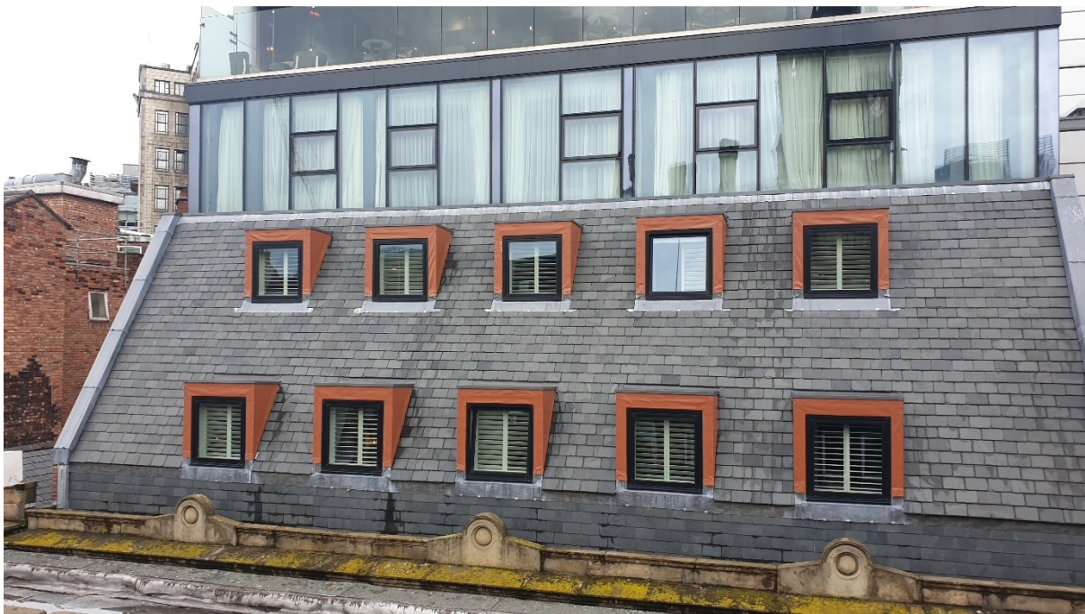
Photograph 1: The south-west aspect of King Street Town House showing the steep pitched slate covered section
