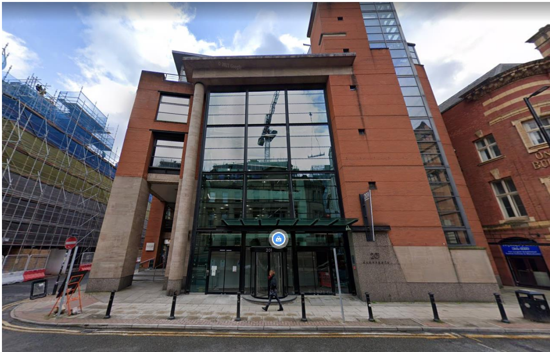
FIGURE 1: EXISTING ELEVATION IMAGE
