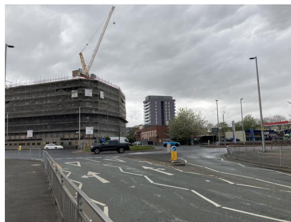
Figure 2.3: View from Higher Ardwick looking south west towards the site, the Polygon St development
