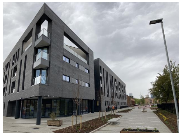
Figure 2.9: View of the Brunswick Village scheme from Brunswick Street.
