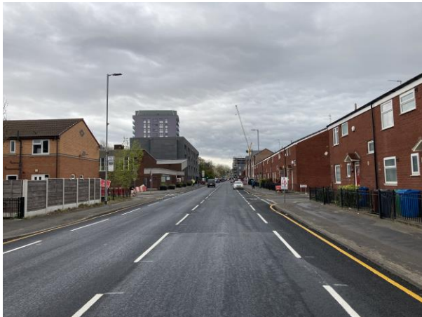
Figure 2.12: View along Brunswick Street from close to Kincardine Road looking north east towards the A6 roundabout.
