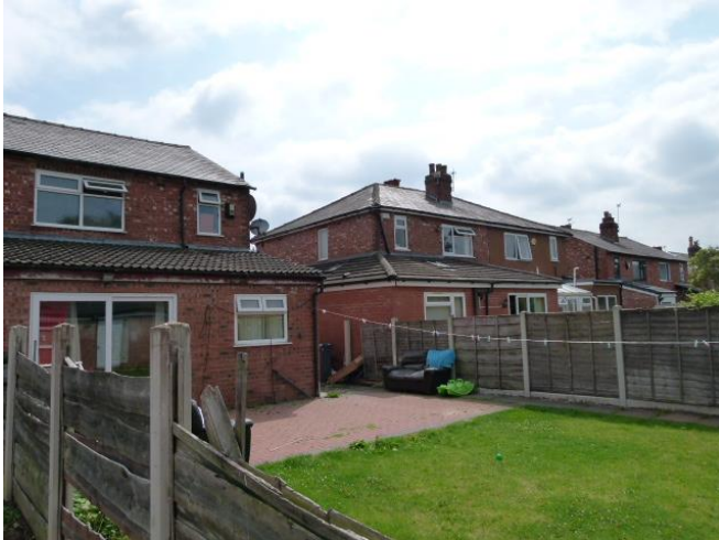
Each application site and the relationship to adjacent properties; No.46 (left) and No.40 (right)
