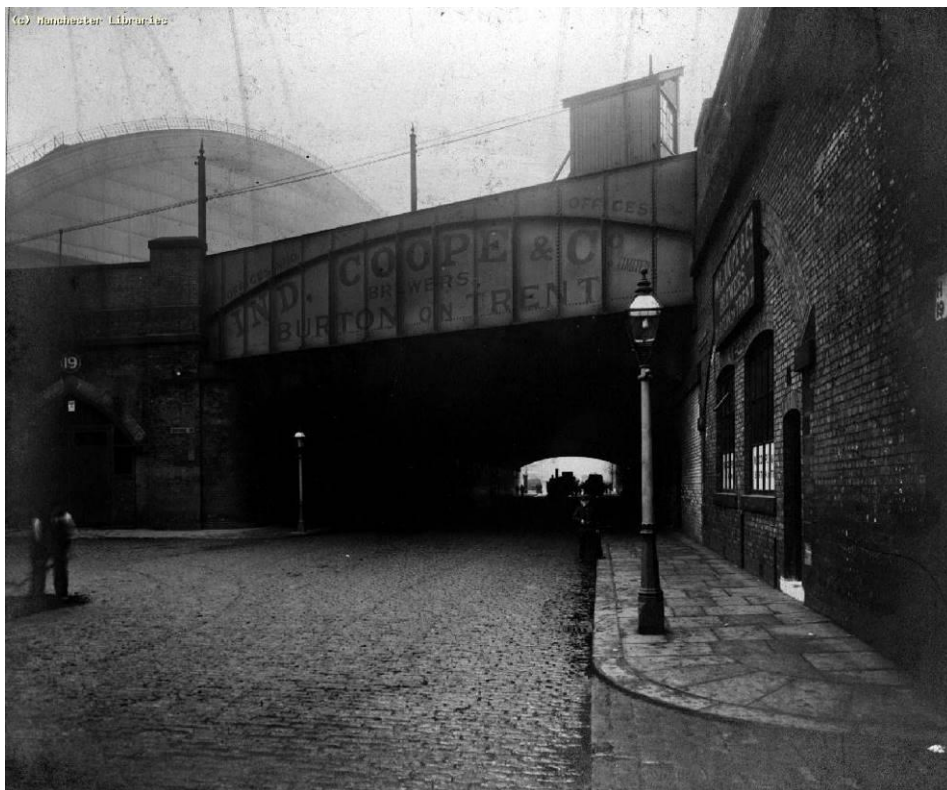
Figure 3: 1909 – A view of the western end of the viaduct at its junction with Watson Street to the left. Note the rear elevation of the former Manchester Central Station to the left of the view.
