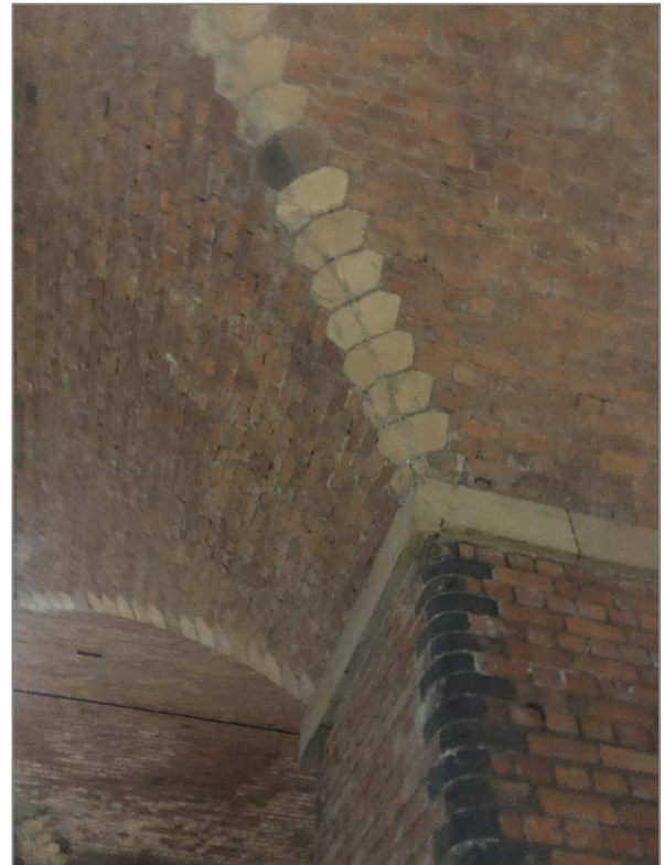
Figures 4 and 5: Site Images (taken 26 th August 2020) from within the Viadux Site illustrating the open character of the space. The historic vaulted ceiling is apparent, supported by large red brick piers and stone quoins. Blue engineering brick provides some detail to the corners of the piers. Note, the Phase 1 works were currently underway in line with the consented scheme.
