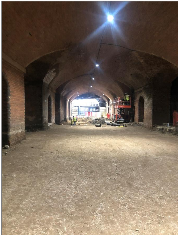
Figures 4 and 5: Site Images (taken 26 th August 2020) from within the Viadux Site illustrating the open character of the space. The historic vaulted ceiling is apparent, supported by large red brick piers and stone quoins. Blue engineering brick provides some detail to the corners of the piers. Note, the Phase 1 works were currently underway in line with the consented scheme.
