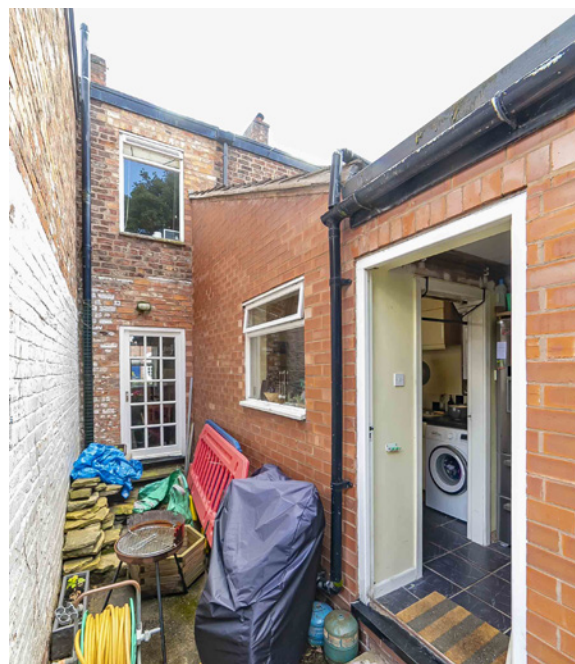
Existing access to garden from living spaces
