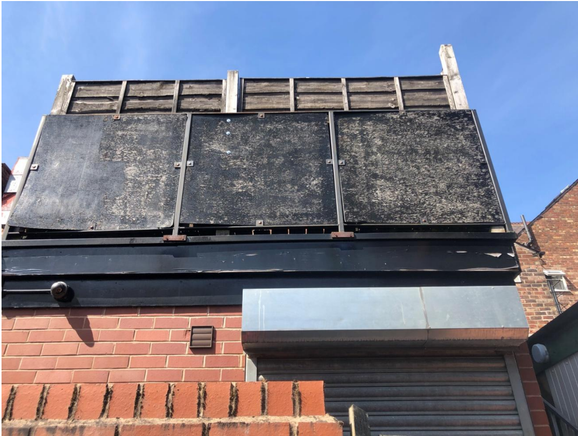
Above: Existing rear elevation
