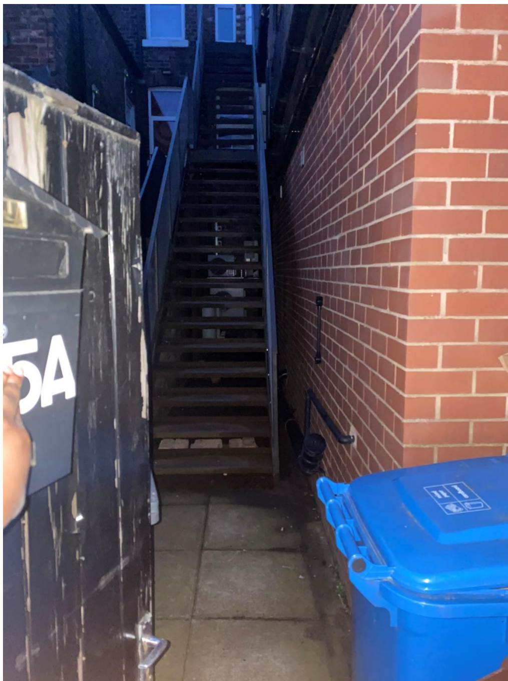
Above: Rear fire escape
