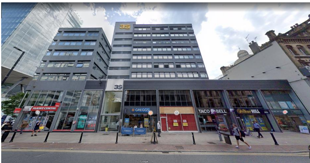
Figure 2: Principal west facing elevation of 39 Deansgate.
