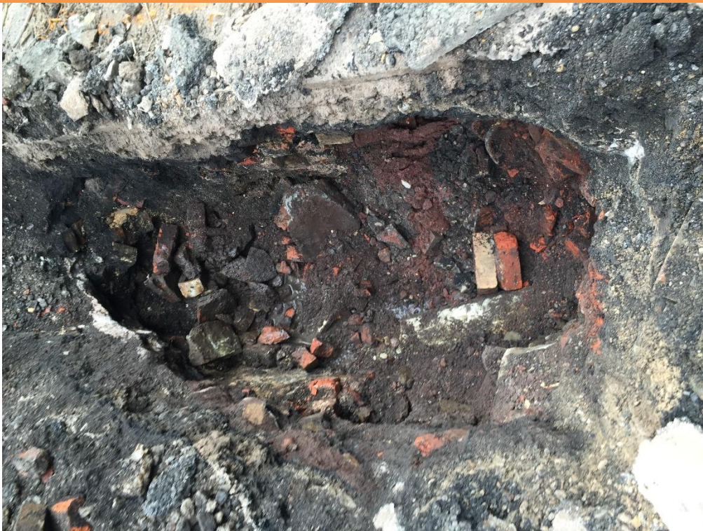
PLATE 8: VIEW OF THE GENERIC MADE GROUND ACROSS THE SITE (TP101)
