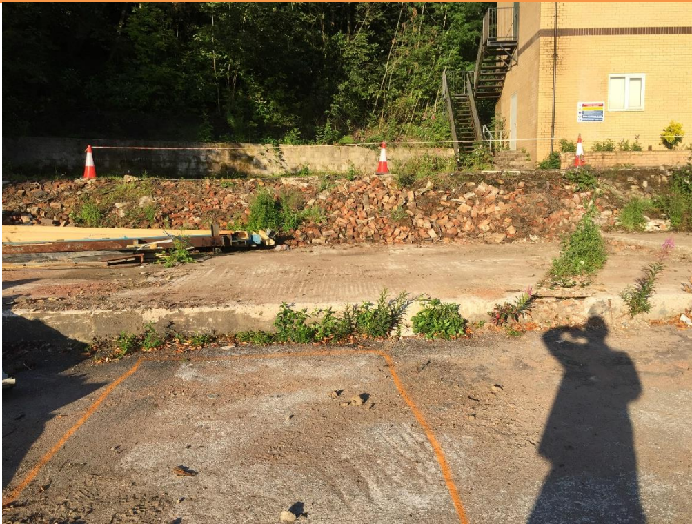
PLATE 7: VIEW OF A REMNANT CONCRETE BUND IN THE SOUTH CENTRAL SECTOR
