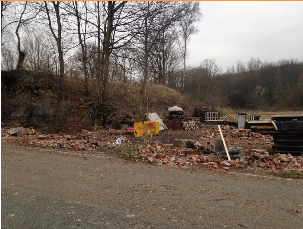
PLATE 3 – VIEW OF THE RETAINING STRUCTURE AND EARTH EMBANKMENT WHICH SEPERATES THE RESERVOIR (WEST) AND CONCRETE SLAB (EAST).
