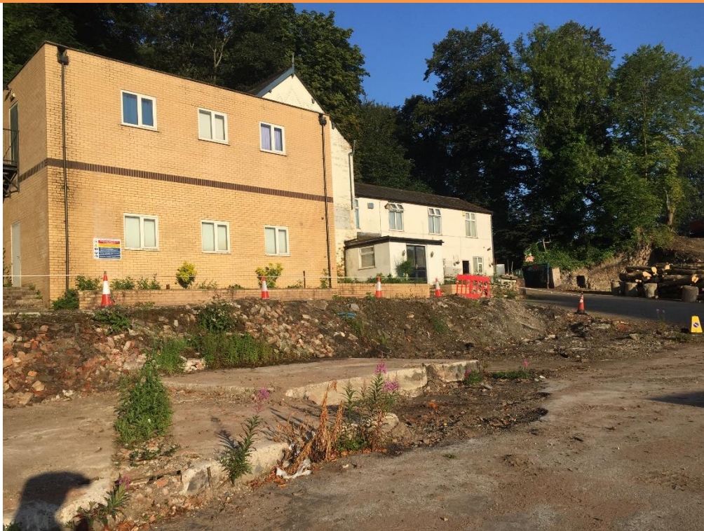
PLATE 6: VIEW OF THE FORMER SITE OFFICE IN THE SOUTH CENTRAL SECTOR
