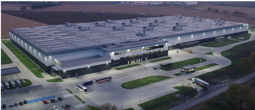
THG Warehouse, Poland
