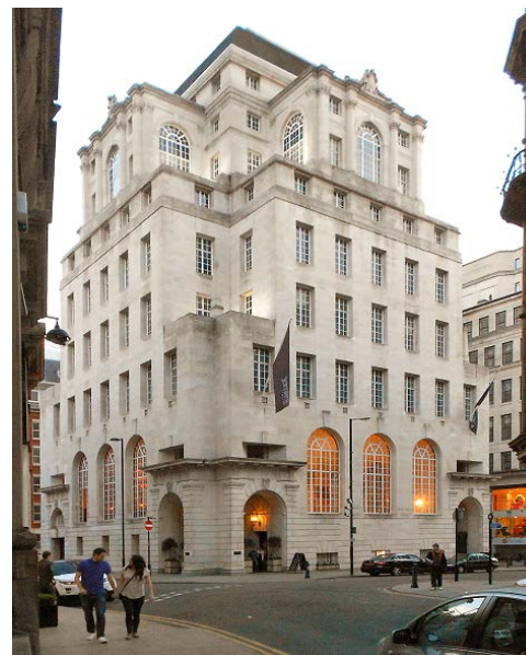
Former Midland Bank at 100 King Street
