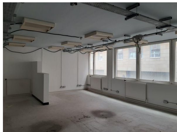
Plate 4.13: Office Space on First Floor.
