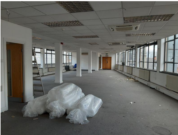
Plate 4.19: Office Space on 6 th Floor of Grange House.
