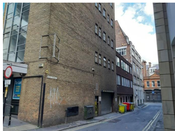
Plate 4.16: Eastern Elevation of Grange House.
