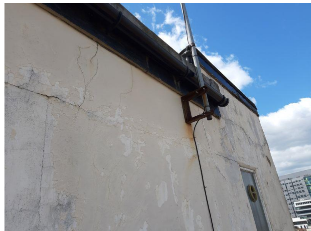
Plate 4.4: External View of Lift Motor Room on Roof of Old Colony.
