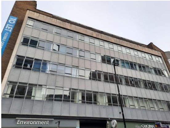
Plate 4.26: Building B3 (Grange House) 17.02.21.
