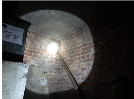
Plate 4.22: Mezzanine Area within Lift Motor Room.
