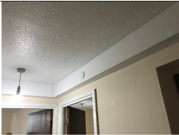
Existing ceilings after sprinkler install
