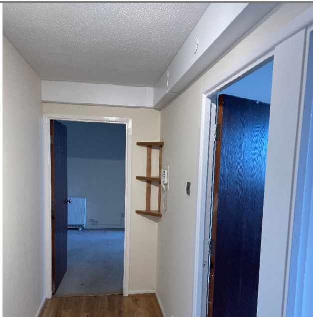
Existing ceilings after sprinkler install
