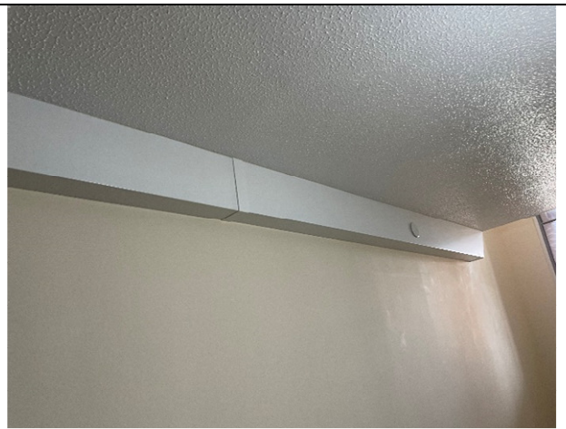
Existing ceilings after sprinkler install
