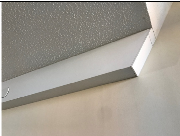
Existing ceilings after sprinkler install
