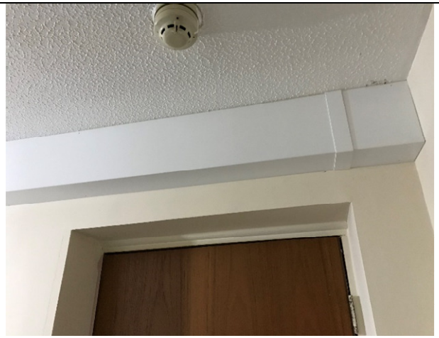
Existing ceilings after sprinkler install
