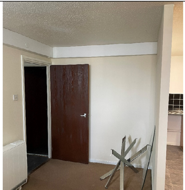
Existing ceilings after sprinkler install
