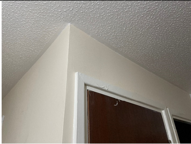
Existing ceilings prior to sprinkler install
