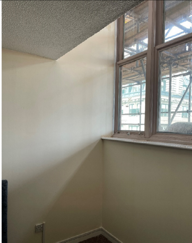
Existing ceilings prior to sprinkler install
