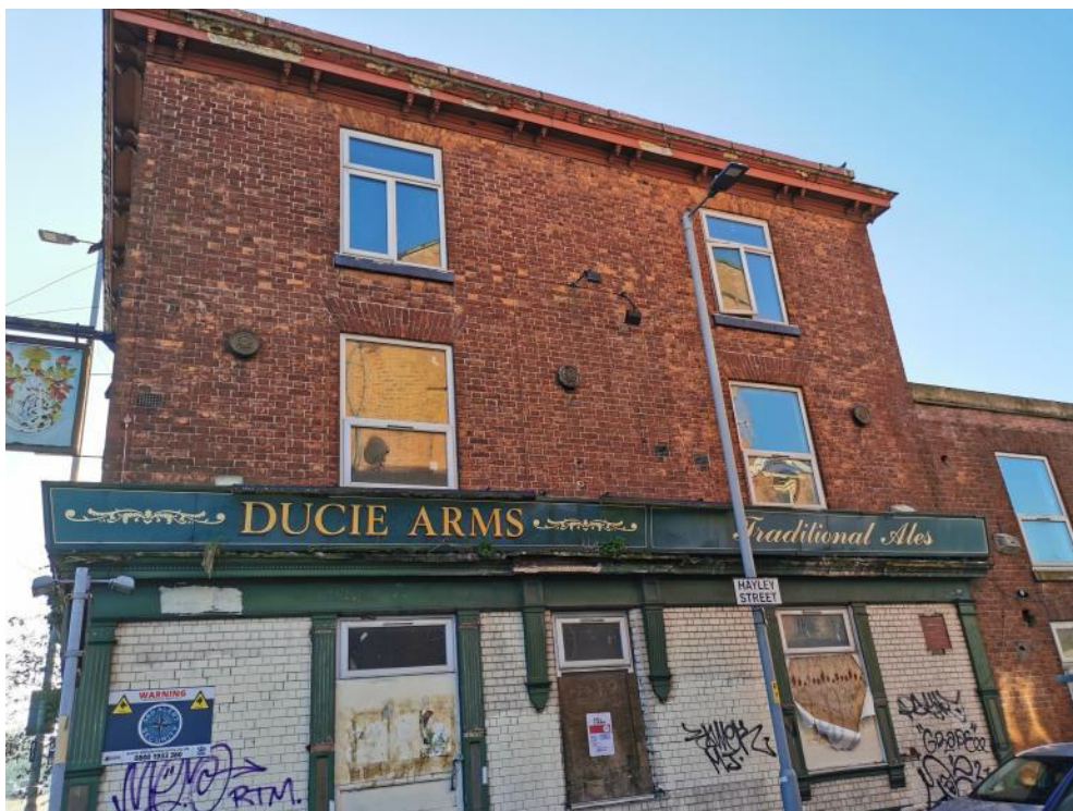
Plate 1 - North-facing elevation of Ducie Arms former public house
