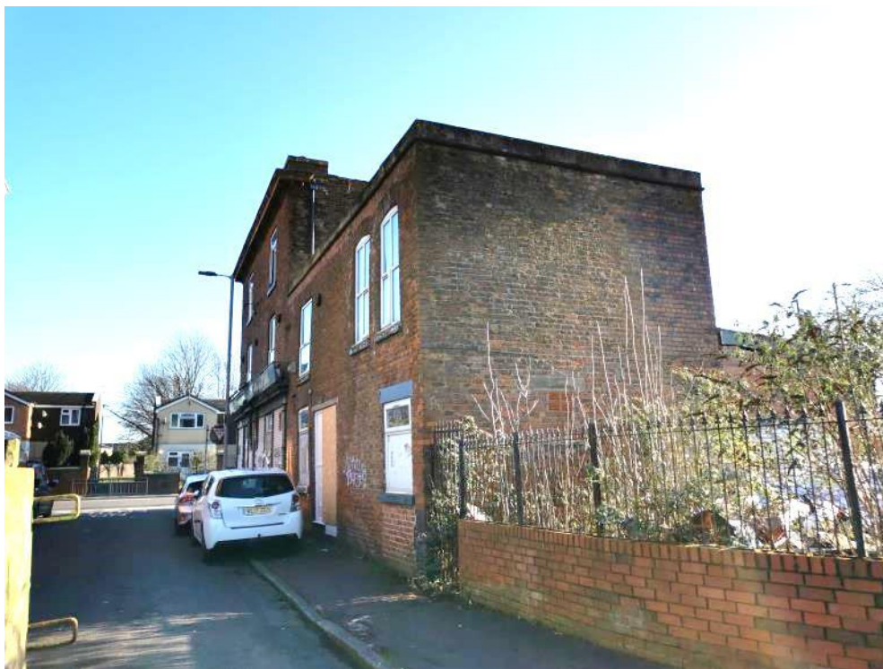
Plate 5 - South-facing elevation of Ducie Arms former public house
