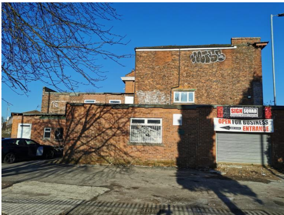
Plate 2 - East-facing elevation of Ducie Arms former public house
