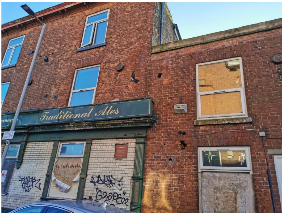
Plate 3 - West-facing elevation of Ducie Arms former public house
