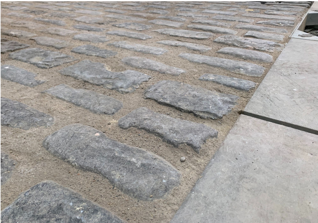
photograph of installed cobble/mortar sample on site
