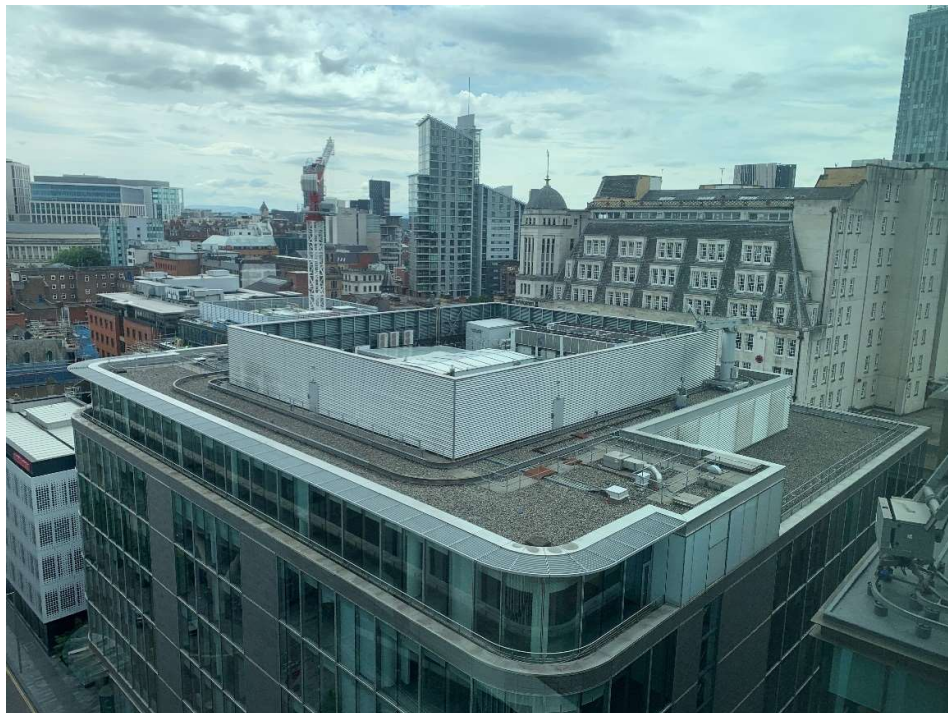
Rooftop Plant Area
