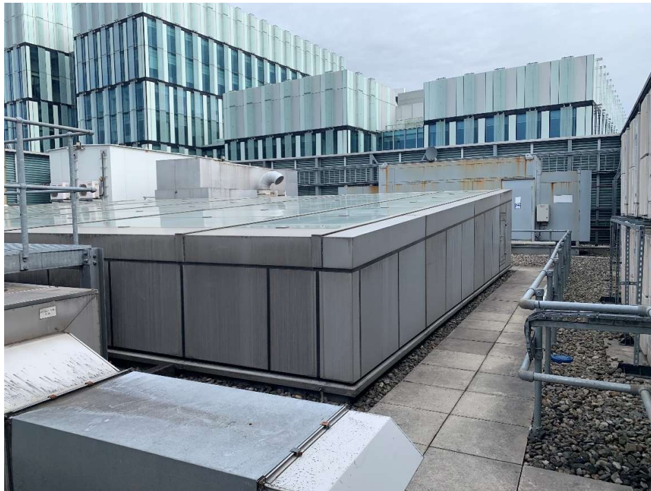
Rooftop Plant Area – Central Atrium and Existing Plant Equipment
