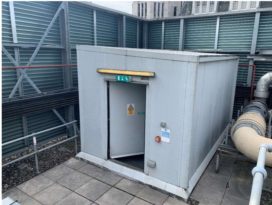
Rooftop Plant Area – Existing Roof Access
