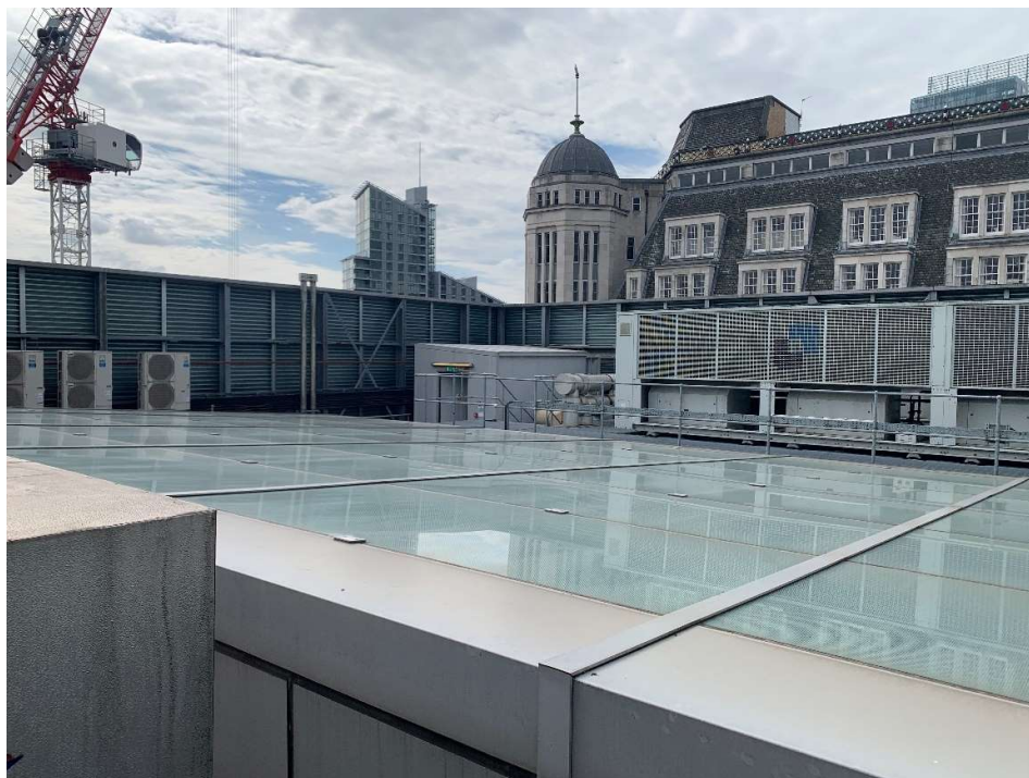
Rooftop Plant Area – Central Atrium, Existing Plant Equipment and Roof Access
