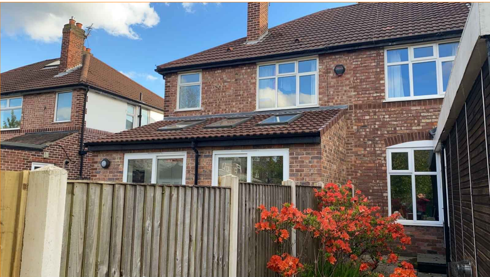
ATTACHED NEIGHBORING PROPERTY REAR
