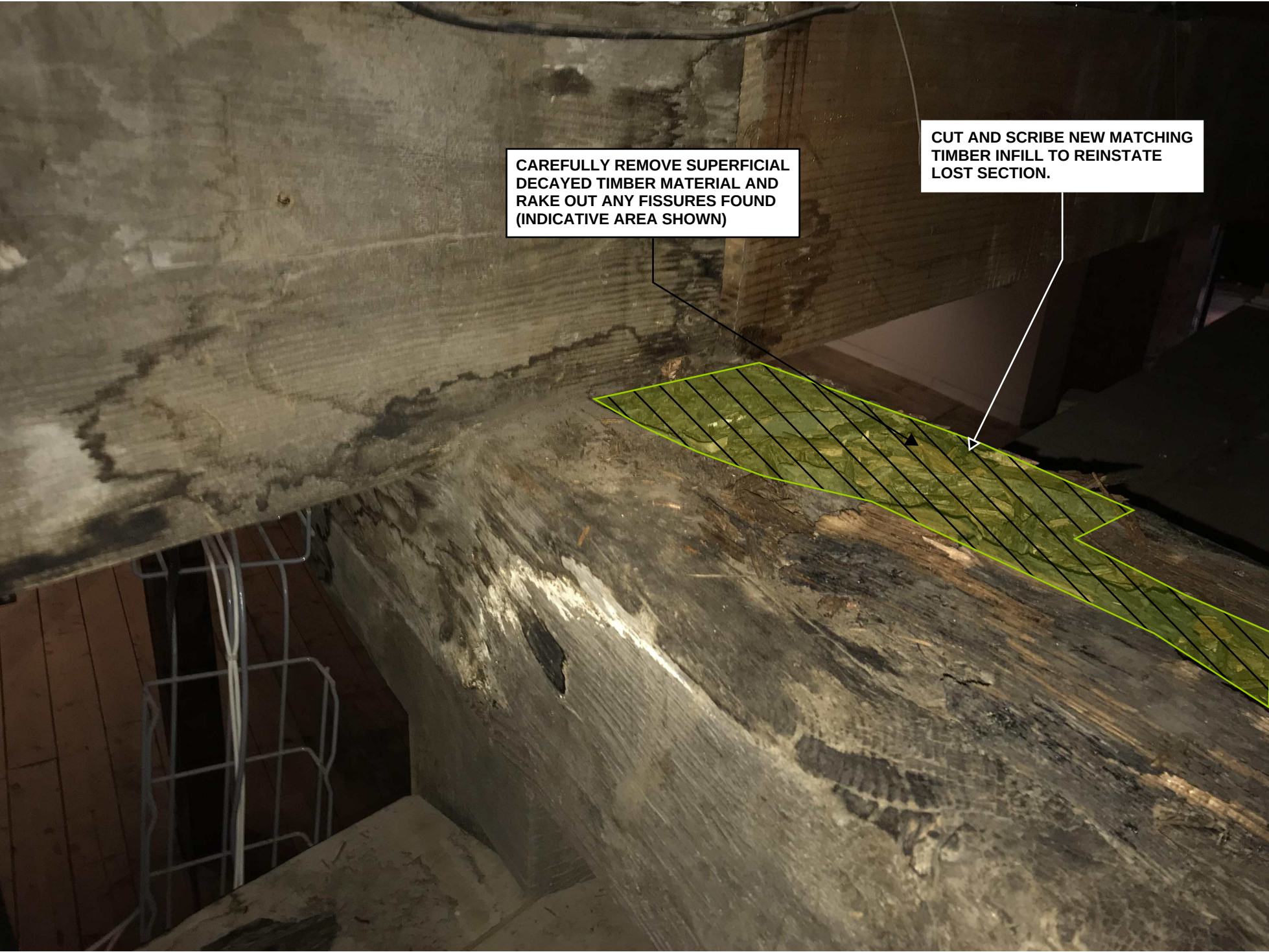
TYPICAL REPAIR FOR SUPERFICIAL TIMBER DECAY
