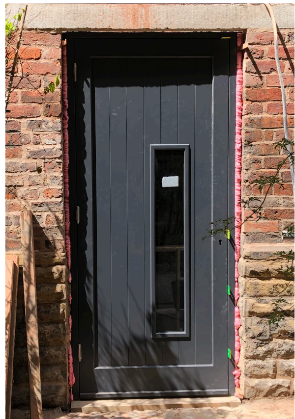
installed timber door on site, pre installation of timber jamb trims 14.07.21
