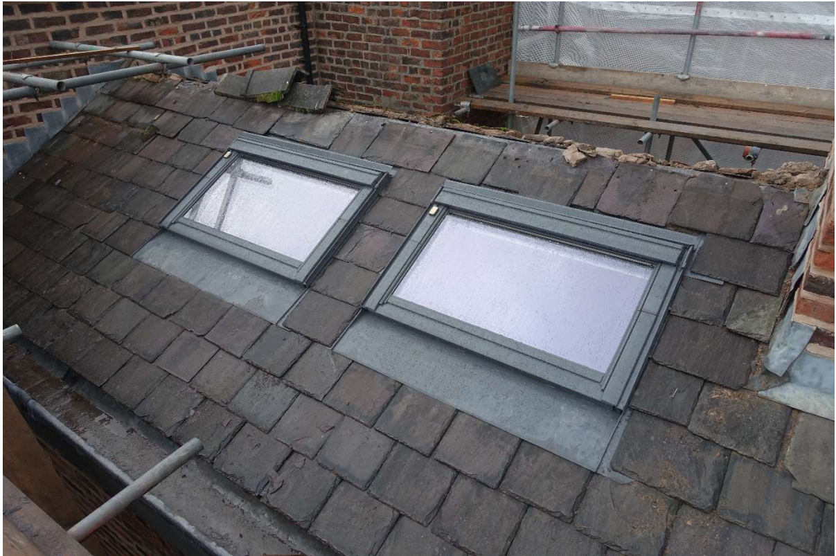
vRear Outrigger Bedroom 5: Existing Rooflight Installation
