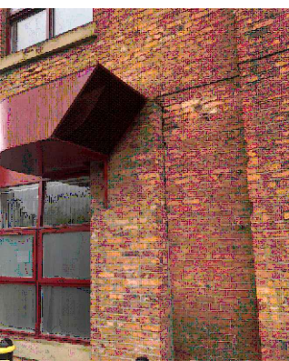
9. Crack between pier and main wall to be repaired with mortar to match existing.
