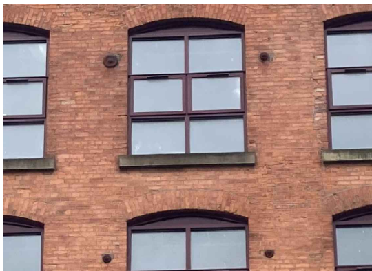
3. Existing metal stabilisation plates to be left in place.
