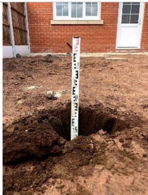
Depth of Cover System at Ground Level
