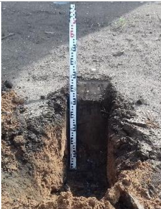
Depth of Cover System at Ground Level
