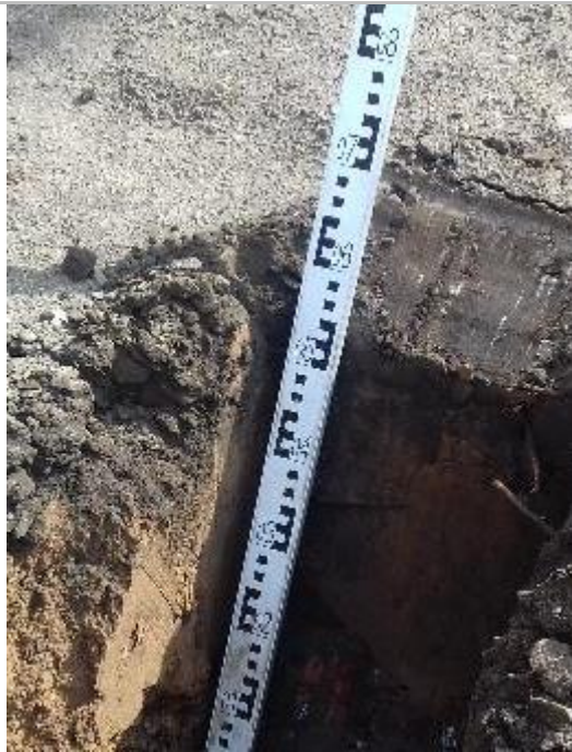
Depth of Cover System at Ground Level
