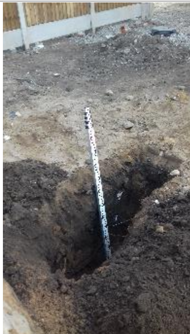
Depth of Cover System at Ground Level
