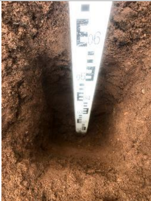
Depth of Cover System at Ground Level
