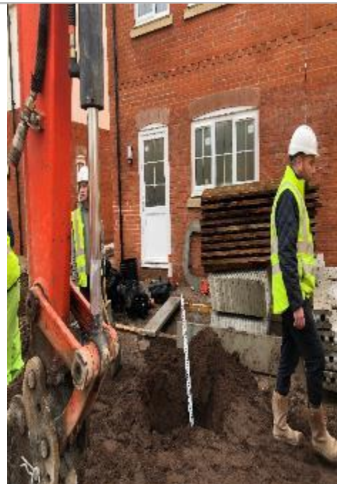
Depth of Cover System in Relation to Plot
