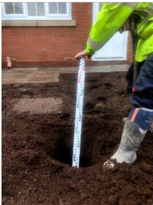
Depth of Cover System at Ground Level
