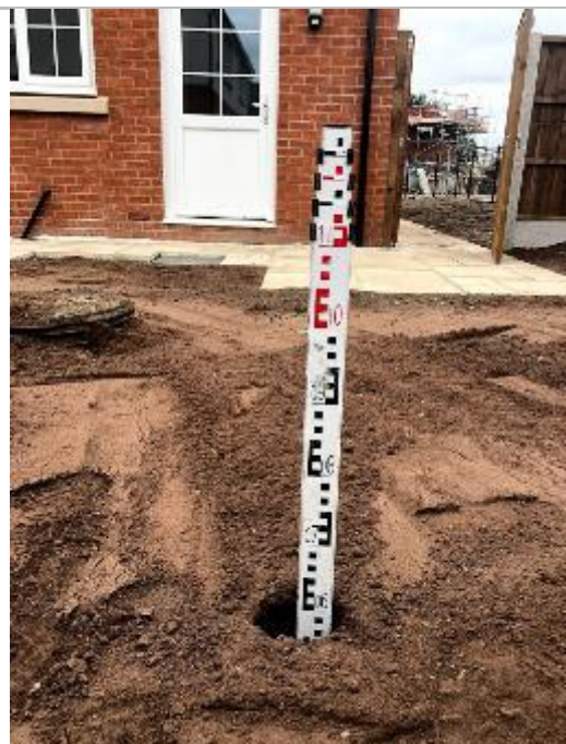
Depth of Cover System at Ground Level
