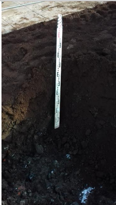
Depth of Cover System at Ground Level
