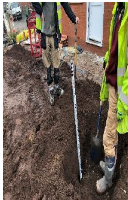
Depth of Cover System in Relation to Plot
