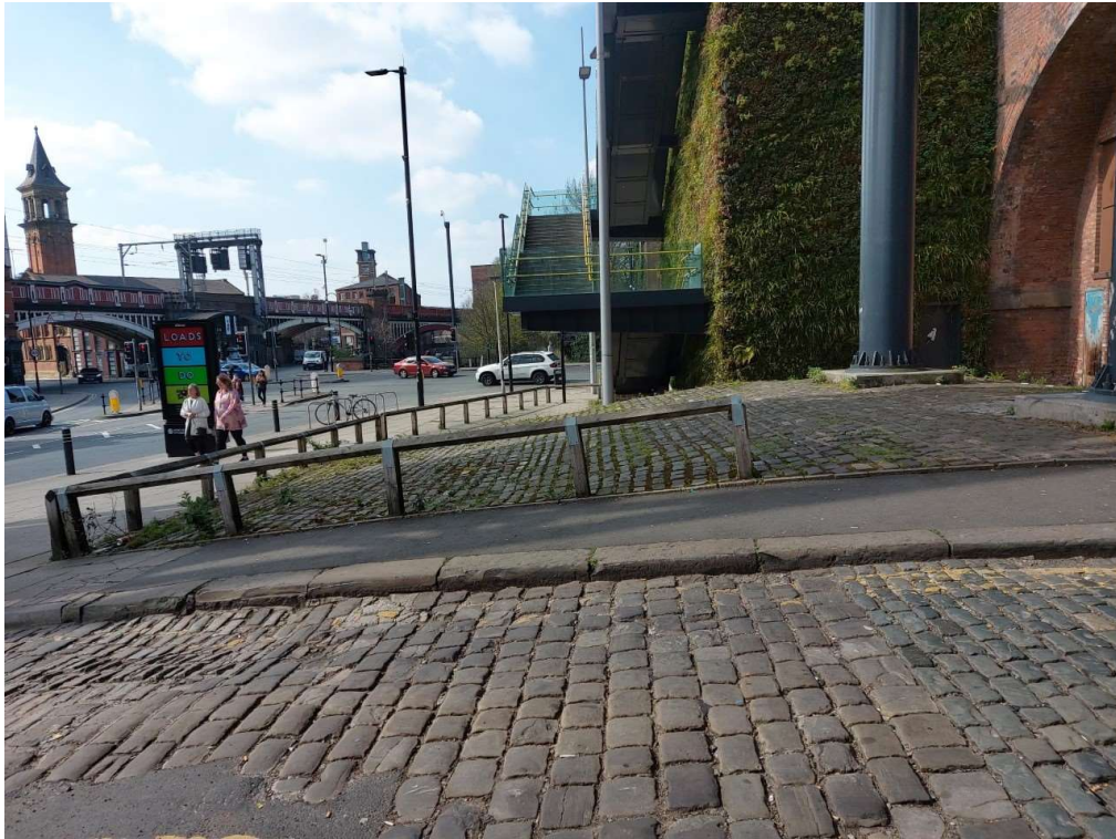
Fig.05 - Image taken from entrance of Lock 91 Bar with Whitworth Street to the left and the listed viaduct to the right. This image demonstrates the site topography and proximity to green wall and staircase to Deansgate Tram Station.
