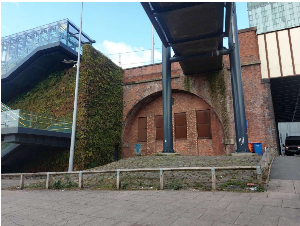
Fig.06 - Image taken from pavement of Whitworth Street directly in front of site and shows the proximity and impact of the green wall and staircase access to Deansgate Tram Station on the site.
