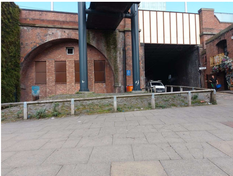
Fig.02 - Image taken from pavement on Whitworth Street directly in front of site showing Lock 91 Bar to the right and green wall to Deansgate Tram Station stair access on the left. Two columns that support the footbridge above are shown falling within the proposed site. Image shows the listed Castlefield Viaduct behind with more recent alterations within the arch.
