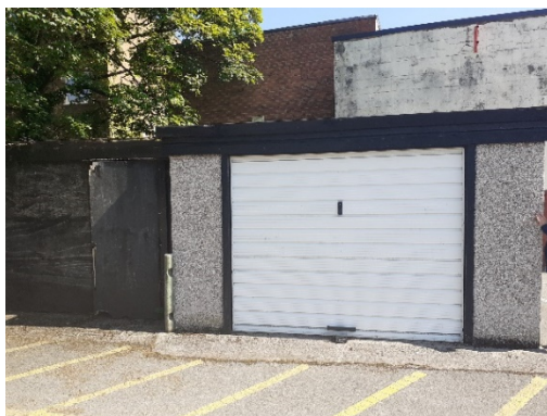
Figure 12: B4 - Garage/shed in rear car park
