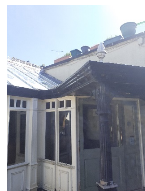
Figure 9: B1 - Rear entrance
