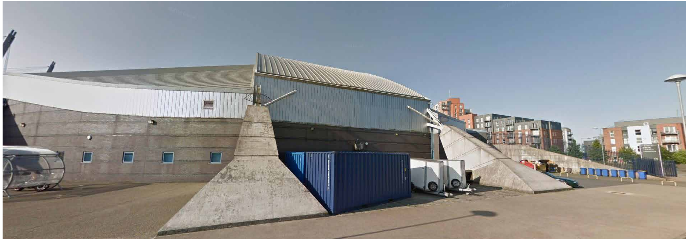
Proposed location of new External plant Area. Taken from the North car park, facing South
