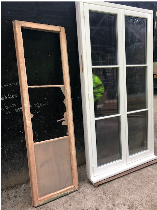
fig01: timber window sample against original pane for comparison as viewed on site. sample provided in white as standard.
