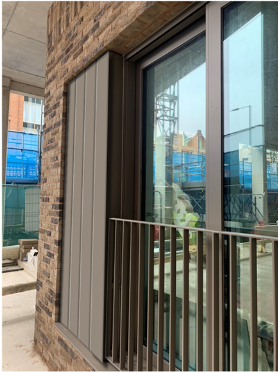
Photograph of On Site Facade Mock Up Panel
