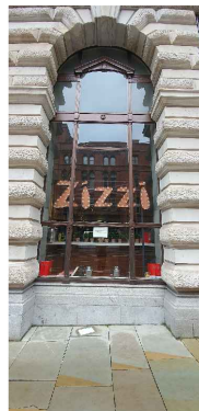
EXISTING SIGNAGE TO BE REMOVED
