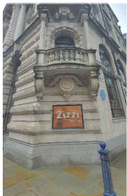
EXISTING SIGNAGE TO BE REPLACED
