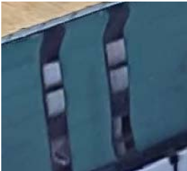
Existing Metal Cladding
