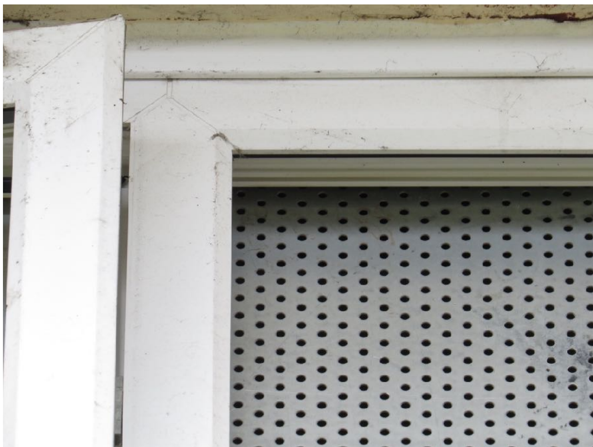
7 – Vacant apartments are secured with steel security panels with no suitable gaps.
