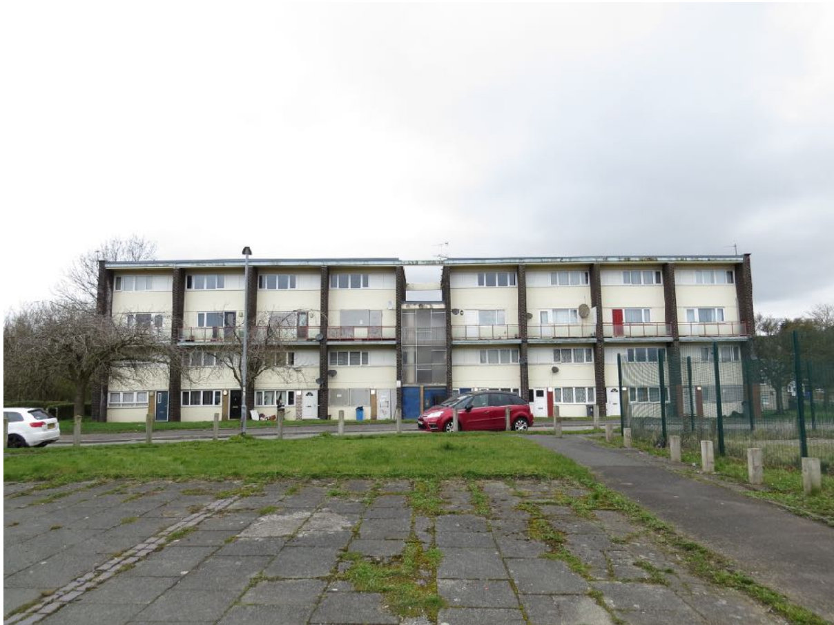
3.1a – The front of the building.
