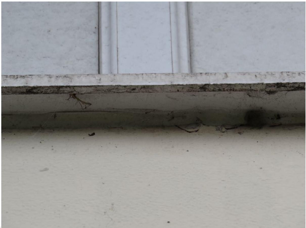
6 – There are no gaps between window and door frames and brickwork.
