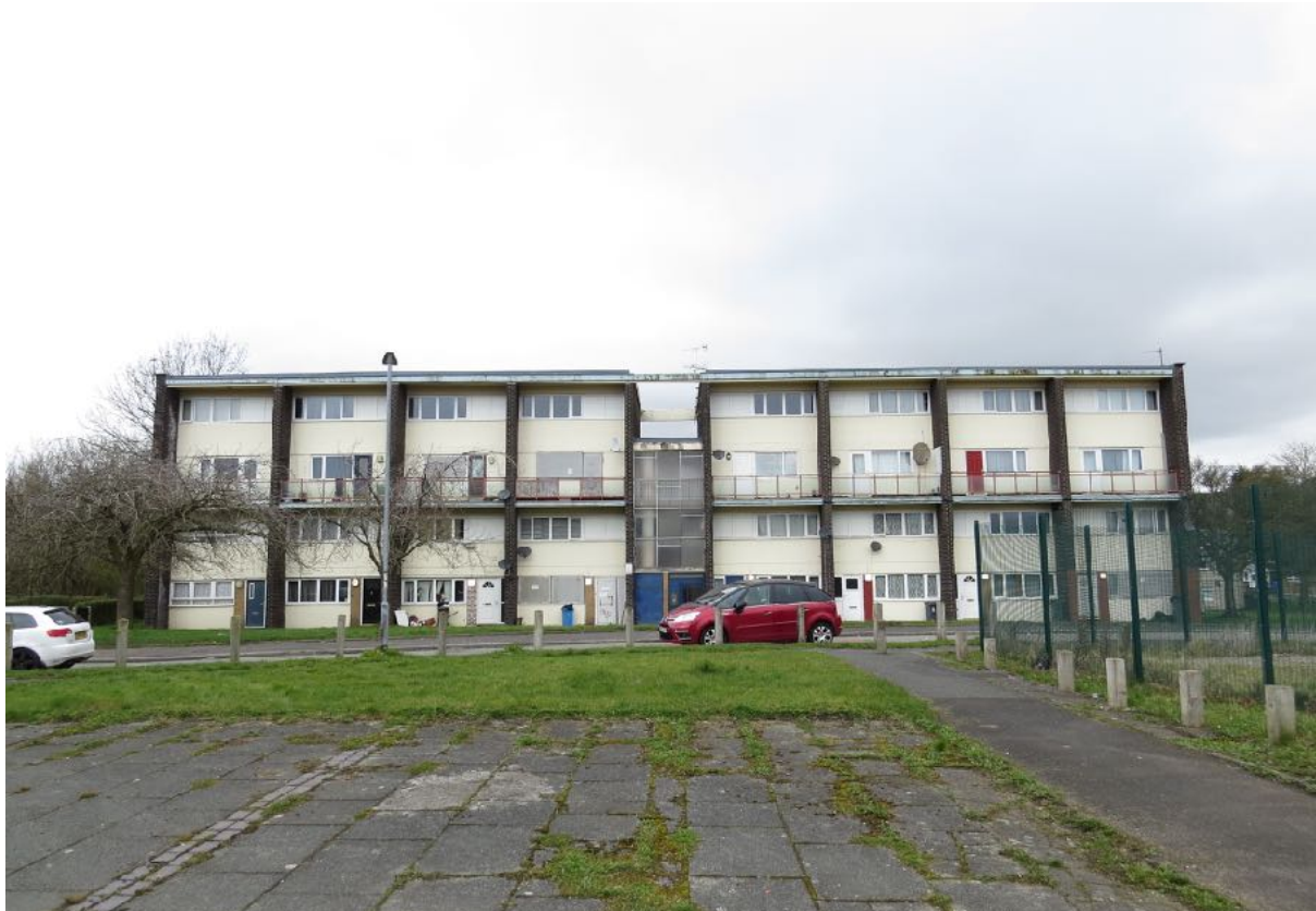
1 – The front of the building.
