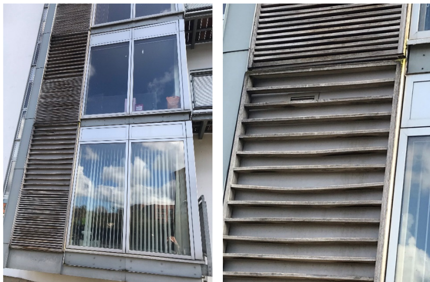
Existing timber louvres
