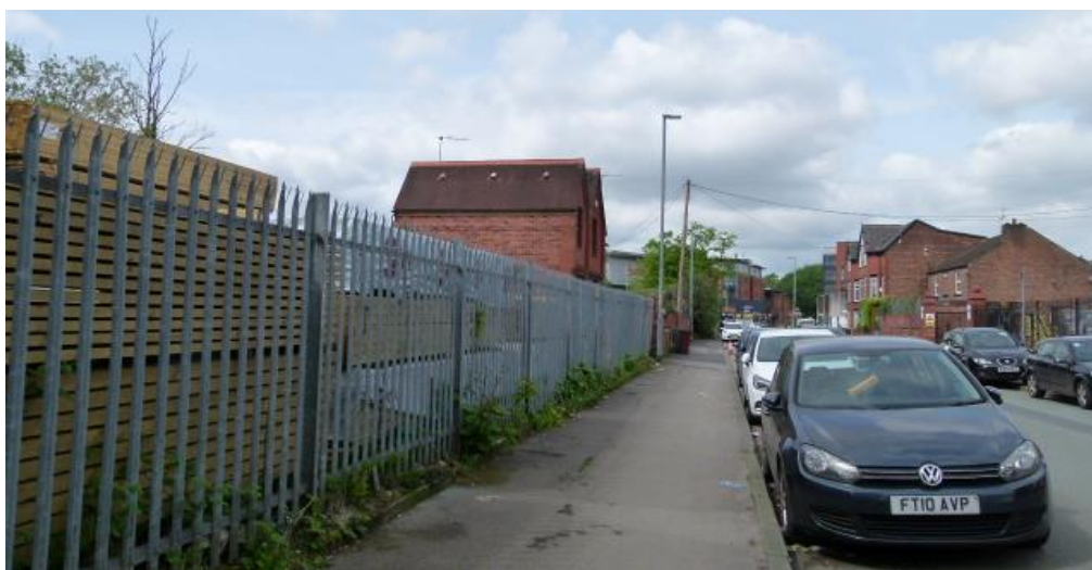
The side elevation as seen from the eastern approach along Ladybarn Road, looking towards Wilmslow Road
