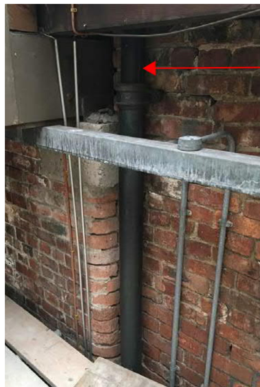
Figure 3-8 - Existing rainwater pipe details
