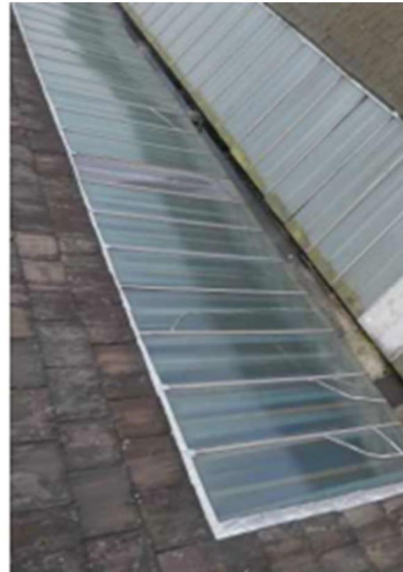
Figure 3-2 - Existing rooflight detail
