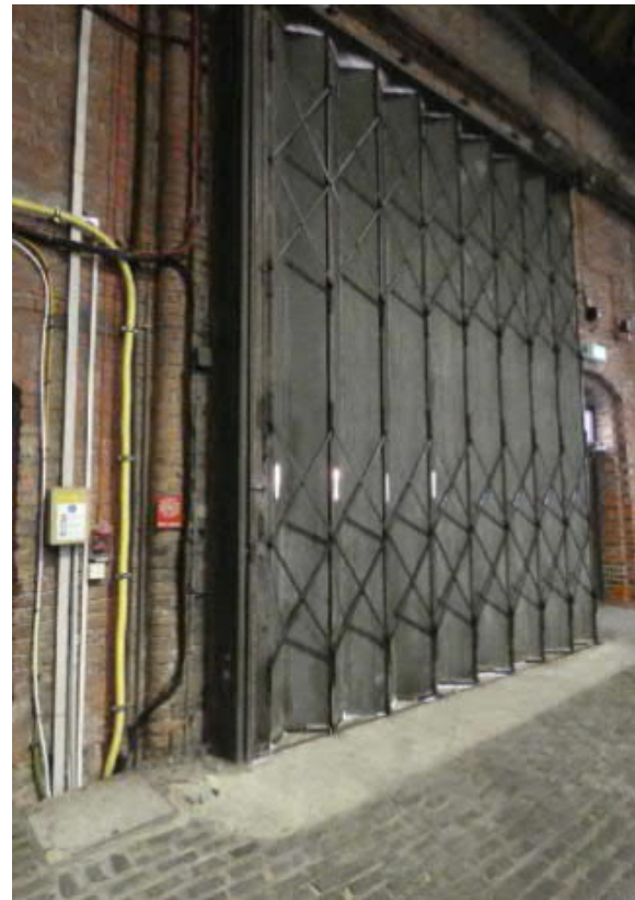
Figure 3-7 - Existing concertina door detail
