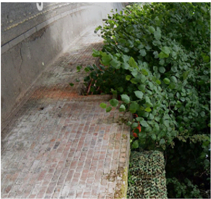
PHOTO 2: CHANGE IN HEIGHT AT END OF WALL
