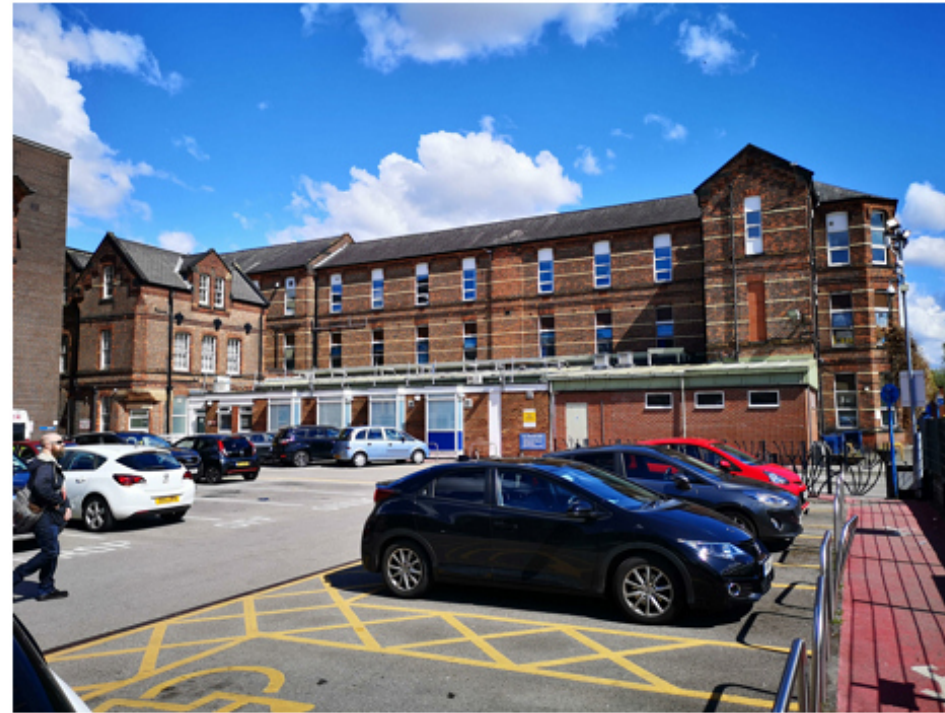
P1 - Photo from Existing Car Park to Endo Suite
