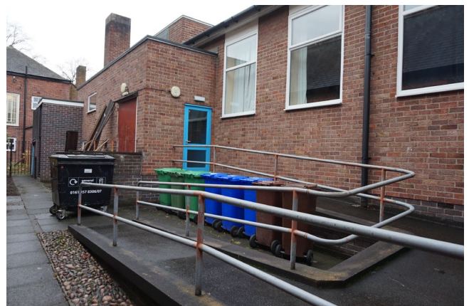
Figure 4: Existing ramp and wheelie bins in the pathway between the buildings.
