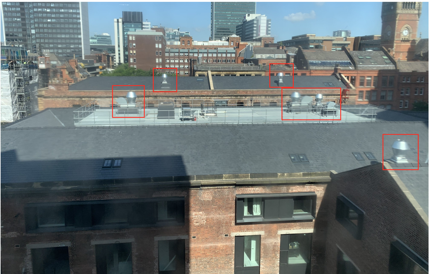
view of minshull + minto rooftops from new build (riser terminations highlighted)
