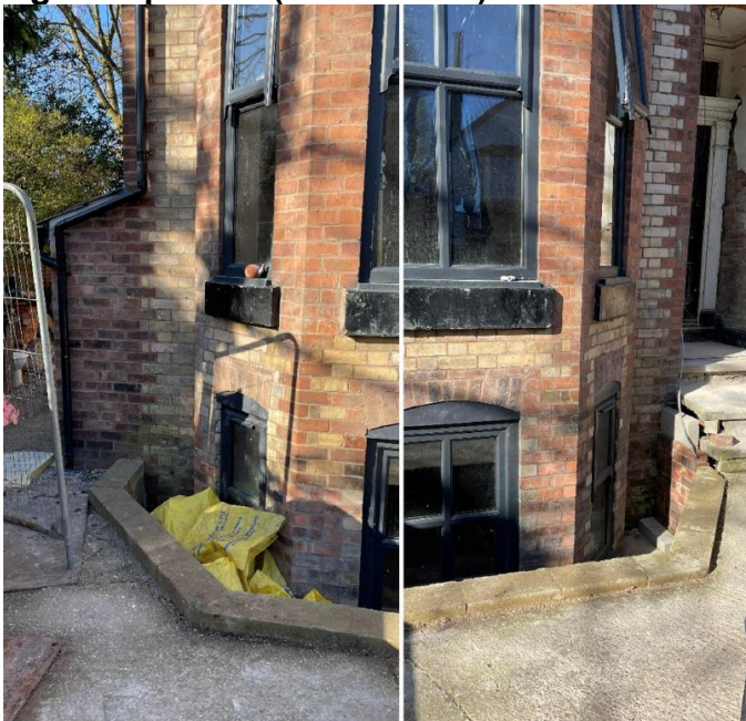
Front elevation with build-out for basement lightwell
