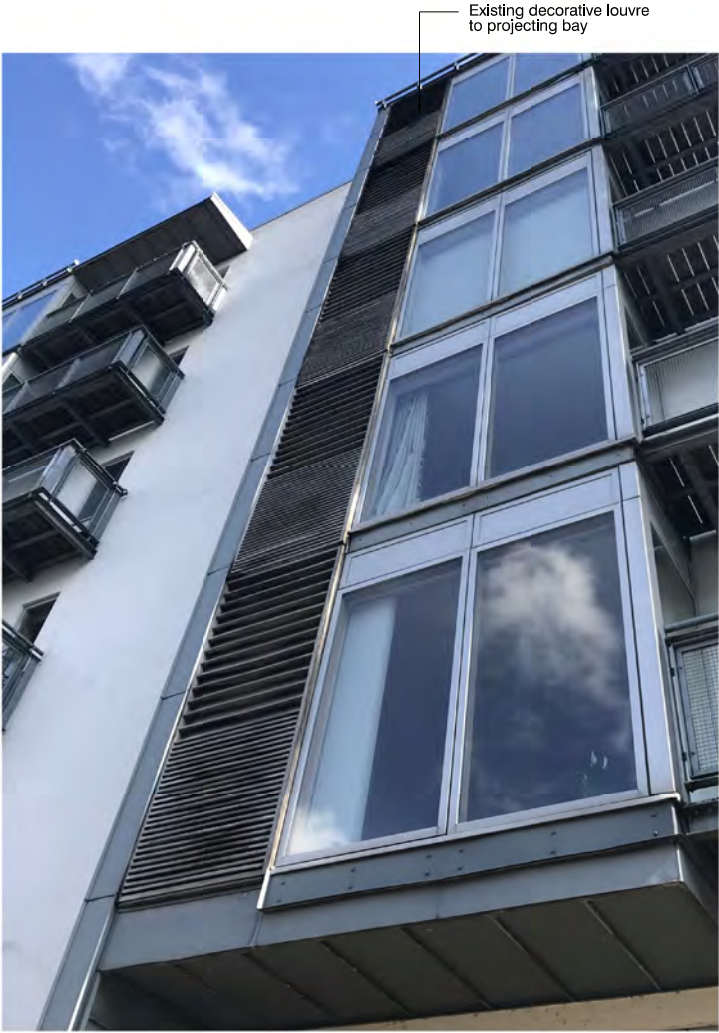
Existing louvre to projecting bays
