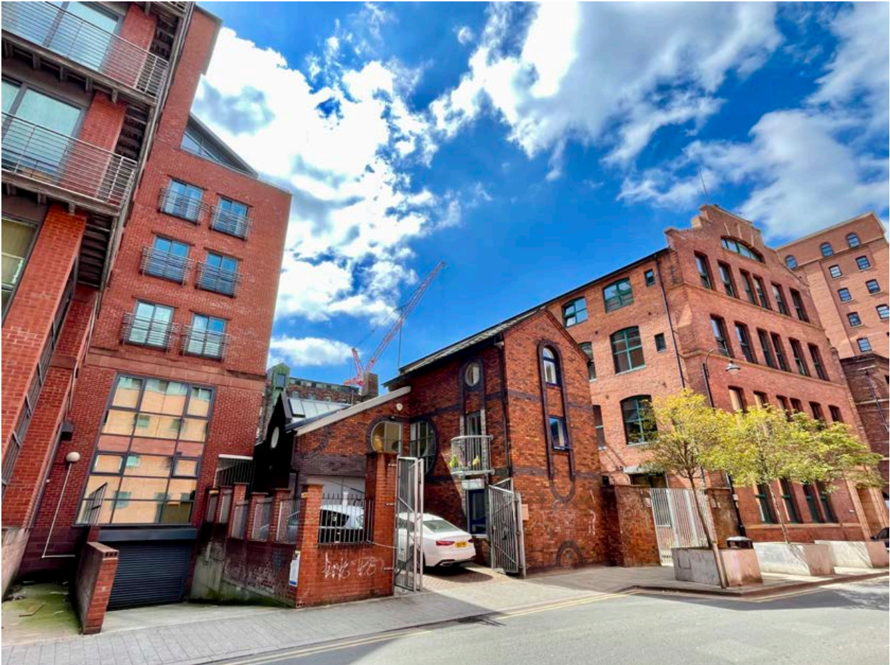
5 Hulme St showing 7 Hulme St to the right and Pearl House to the left.
