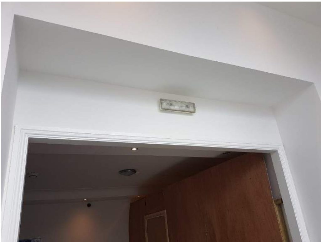
Image 008: Modern architrave to be removed.
