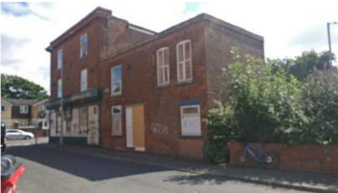
Photograph 2: View facing north east towards the Site
