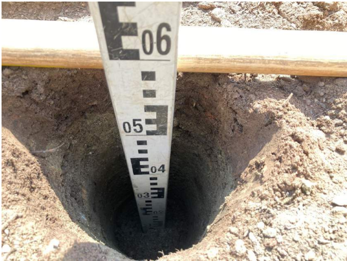
Photograph 5 150mm of topsoil and 450mm of subsoil emplaced in VP03.
