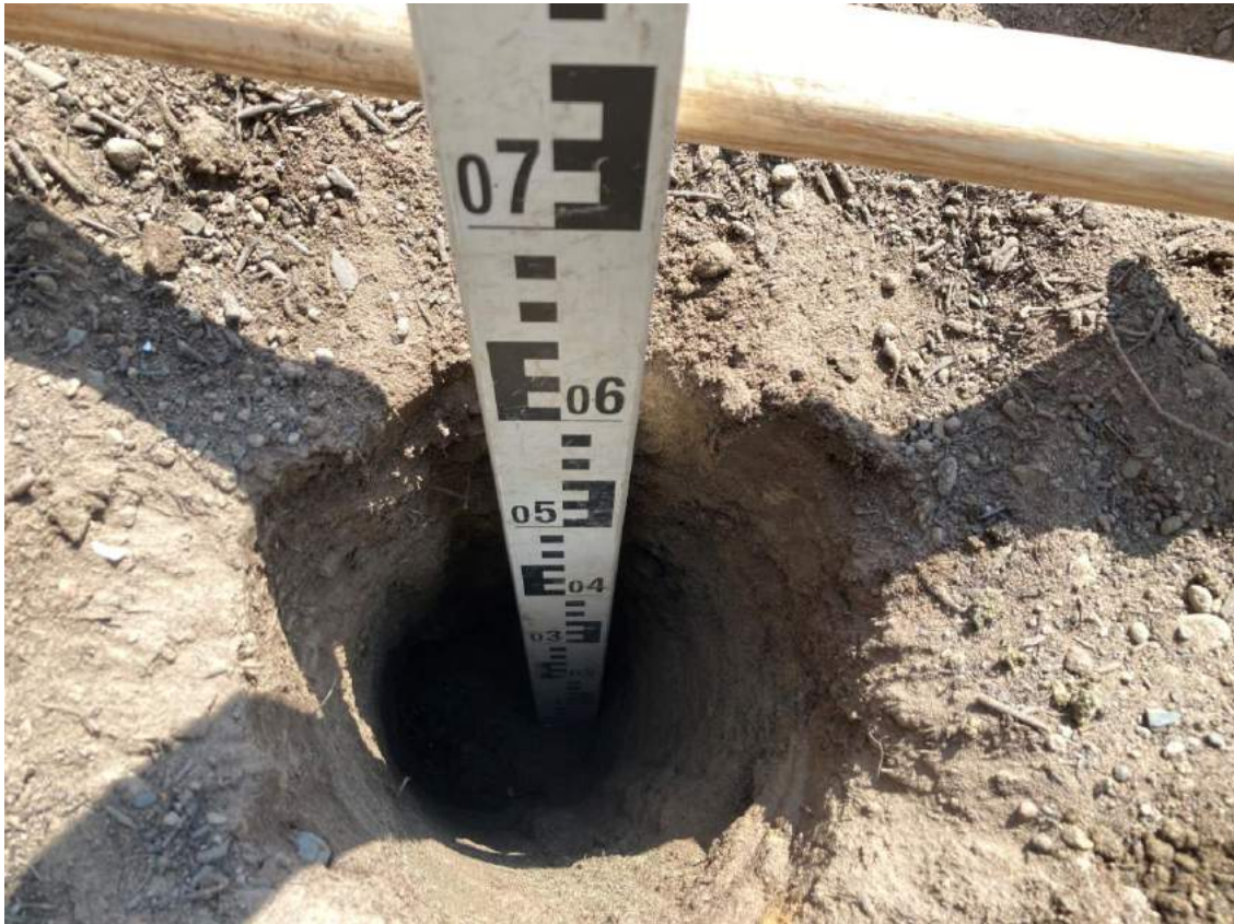
Photograph 3 150mm of topsoil and 450mm of subsoil emplaced in VP02.
