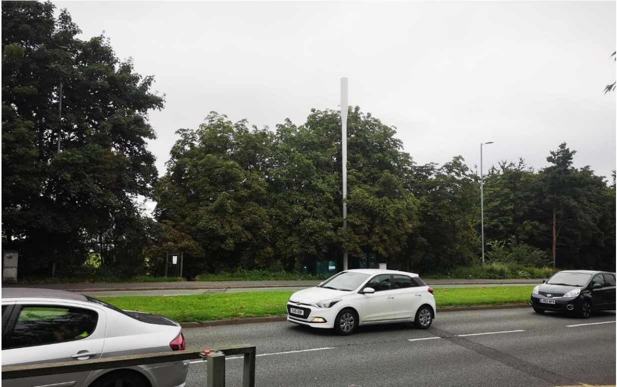
Existing mast - the application proposals would be sited 13m to the right
