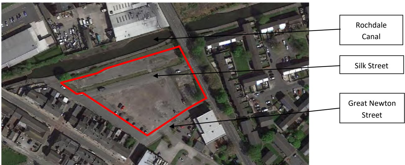
Figure 1: Aerial Photograph of Existing Site (Google, 2021)
