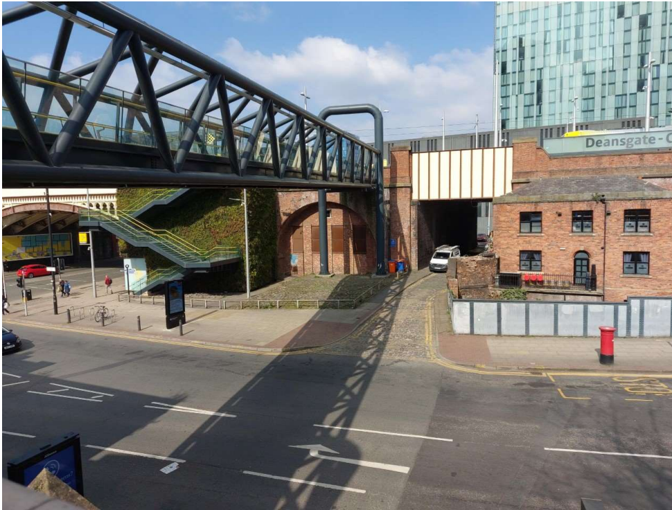
Fig.01 - Image taken from ramped access to Deansgate Station on the south side of Whitworth Street looking north. Image shows Lock 91 Bar on the far right, stair access to Deansgate Tram Station and the proposed site in between with the footbridge directly above. The site is bound by low level timber balustrades on two sides. Photo shows the site's proximity to Whitworth Street and demonstrates that no residential units or commercial premises are located in the vicinity. The only unit is Lock 91 to which this proposal is associated.
