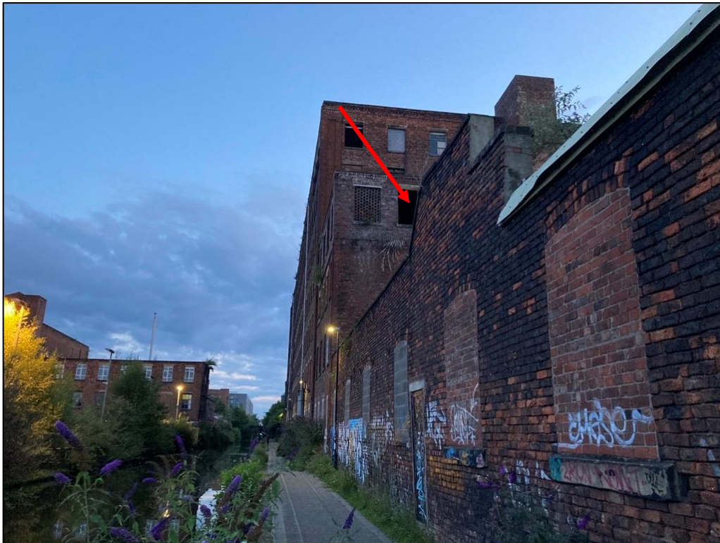
Photograph 1 showing the location of the Common Pipistrelle emergent point (red arrow)
