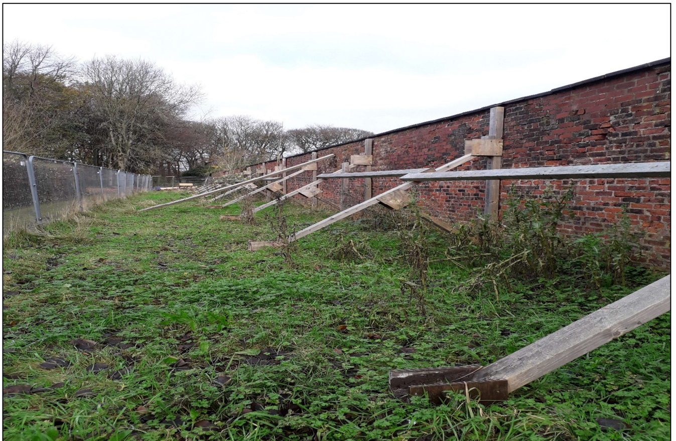
Photo No.2 – View along the West Elevation Boundary Wall to the Horticultural Centre.
