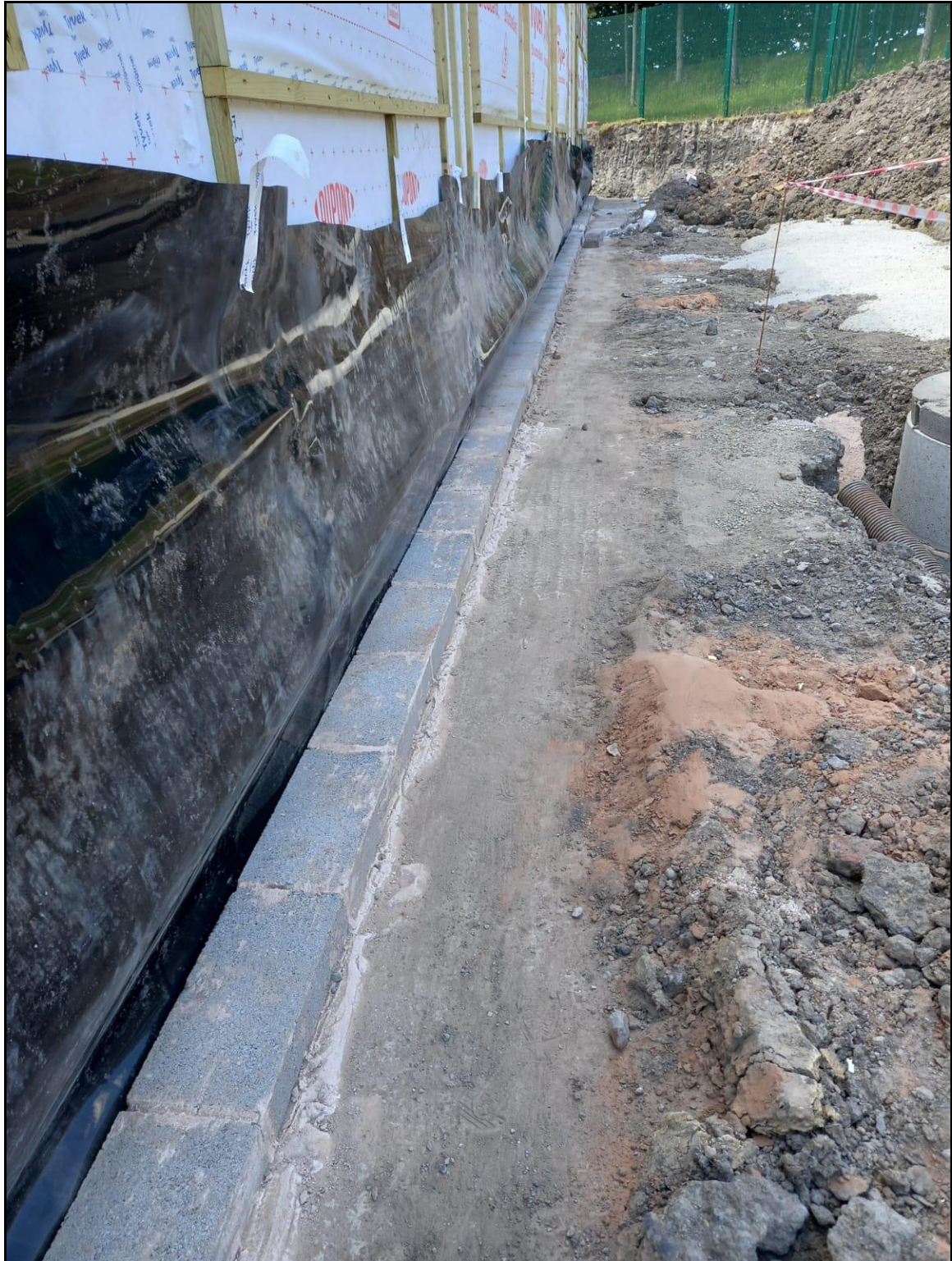
Photograph 5 – Edge detail showing blockwork which was used as formwork for the concrete slab, gas membrane fixed temporarily to the outside of the modules
