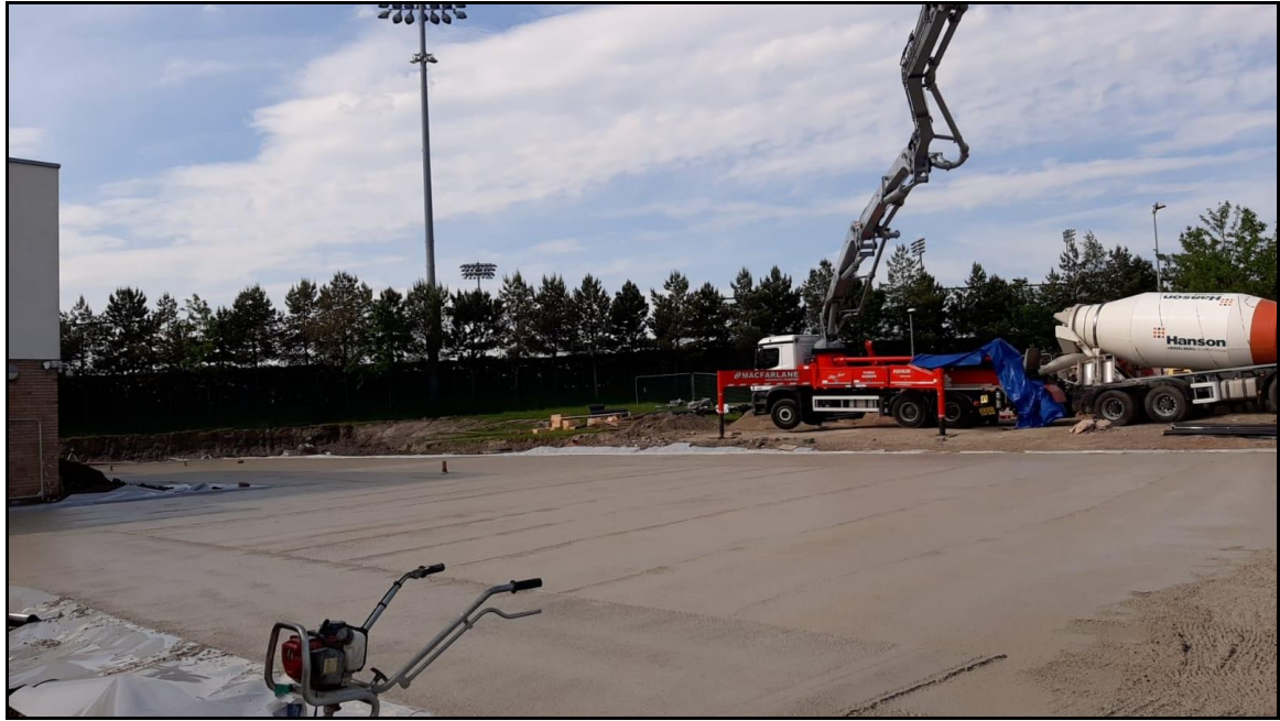
Photograph 4 – Completion of concrete ground bearing slab
