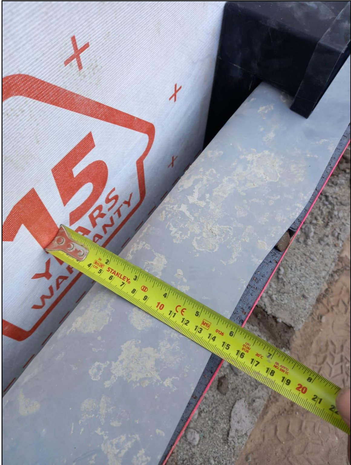
Photograph 7 – Gas barrier onto brick work, note sub-floor vent in top of photograph.
