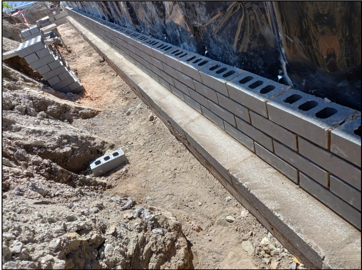
Photograph 6 – Brickwork to gas barrier level
