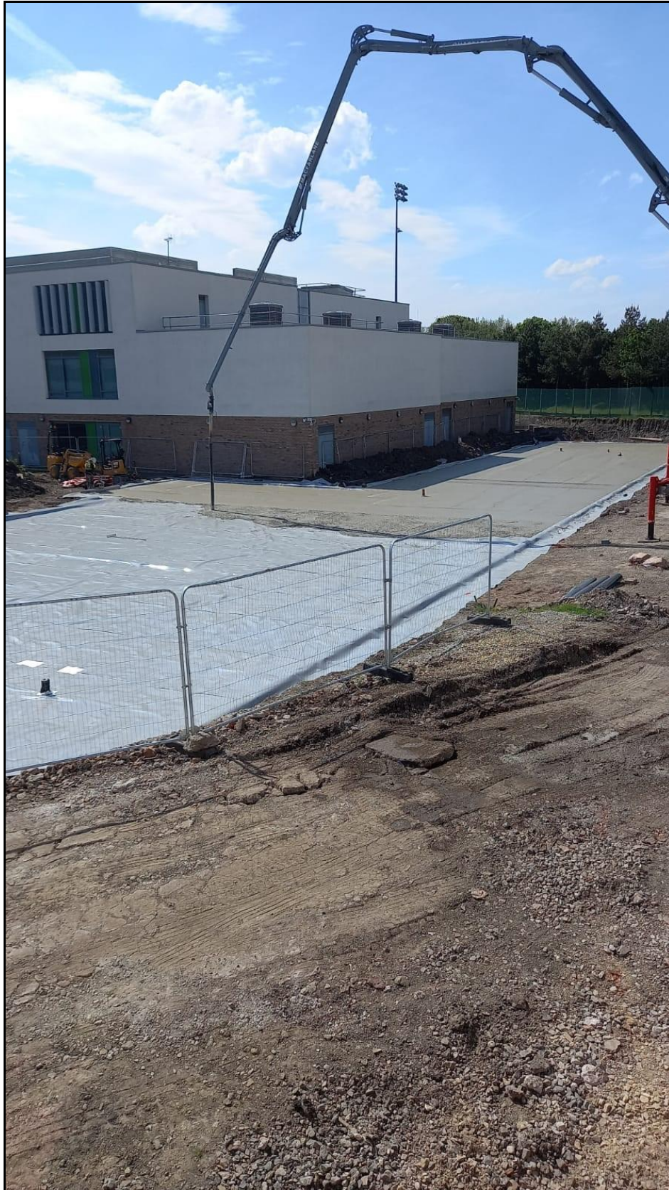
Photograph 3 – installation of concrete ground bearing slab
