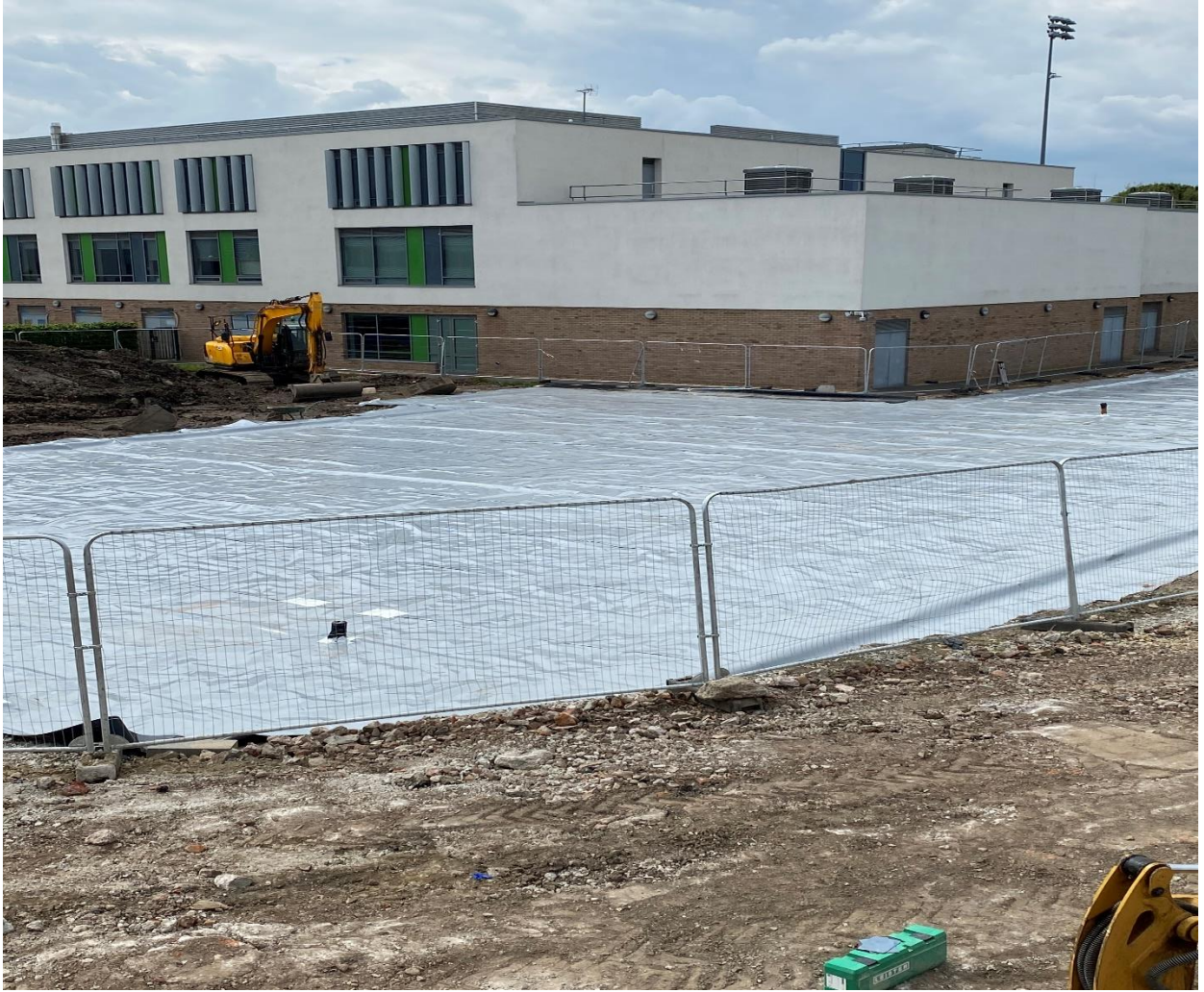
Area overview – 1mtr overlap around entire perimeter to enable it to be lapped onto the modular building
