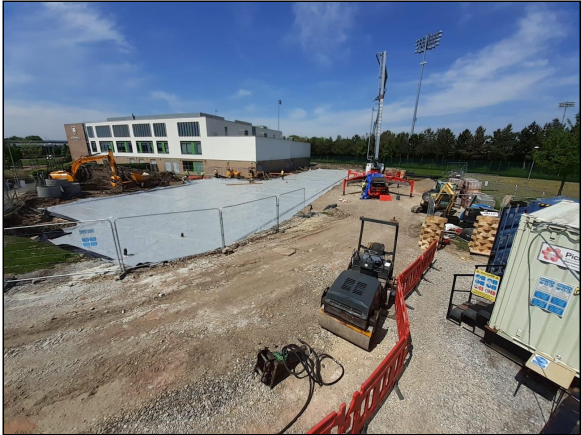
Photograph 1 – View across gas membrane (30/05/21)
